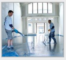
The SP 20 THF is specially designed for liquid screed. In addition a hose decompression is integrated to reduce hose bursts and blockages.
